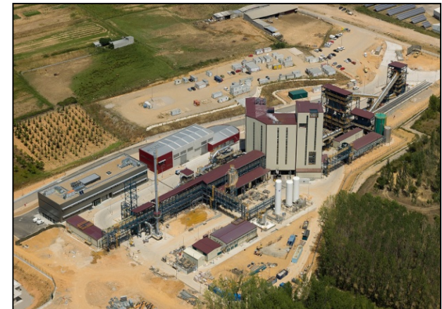
CIUDEN's Technology Development Centre for CO 2 Capture (es.CO 2 )
